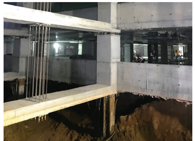
Deep basement excavation level B4
